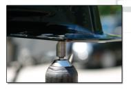
15. Using 1/2" counter sink bit, counter sink the hole on the bottom of the cav plate to fit the supplied mounting bolt.
